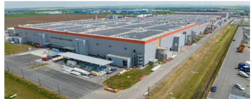
Construction site of CATL in Arnstadt
